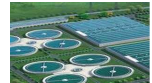
Sewage treatment plants
