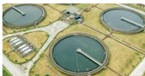
Sewage treatment plants
