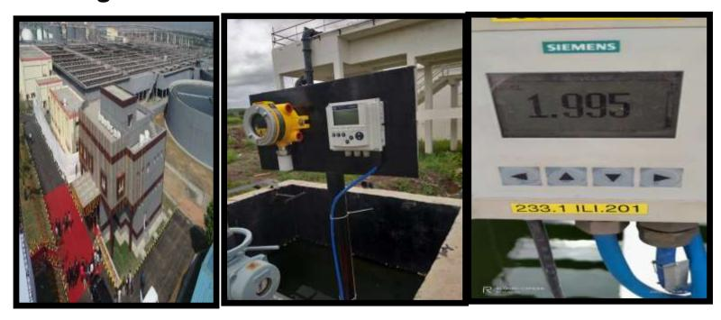
We have installed various analysers like, COD, BOD, TSS, pH, Chlorine, Electromagnetic Flow meters, H2S analyses etc with complete PLC automation and Scada for 5 MLD STP and 6 MLD CETP at Aurangabad. Contractor was Passavat.
