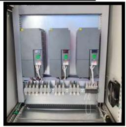
VFD and Soft starter panel with PLC supplied to one of the treatment plant project in Mauritius
